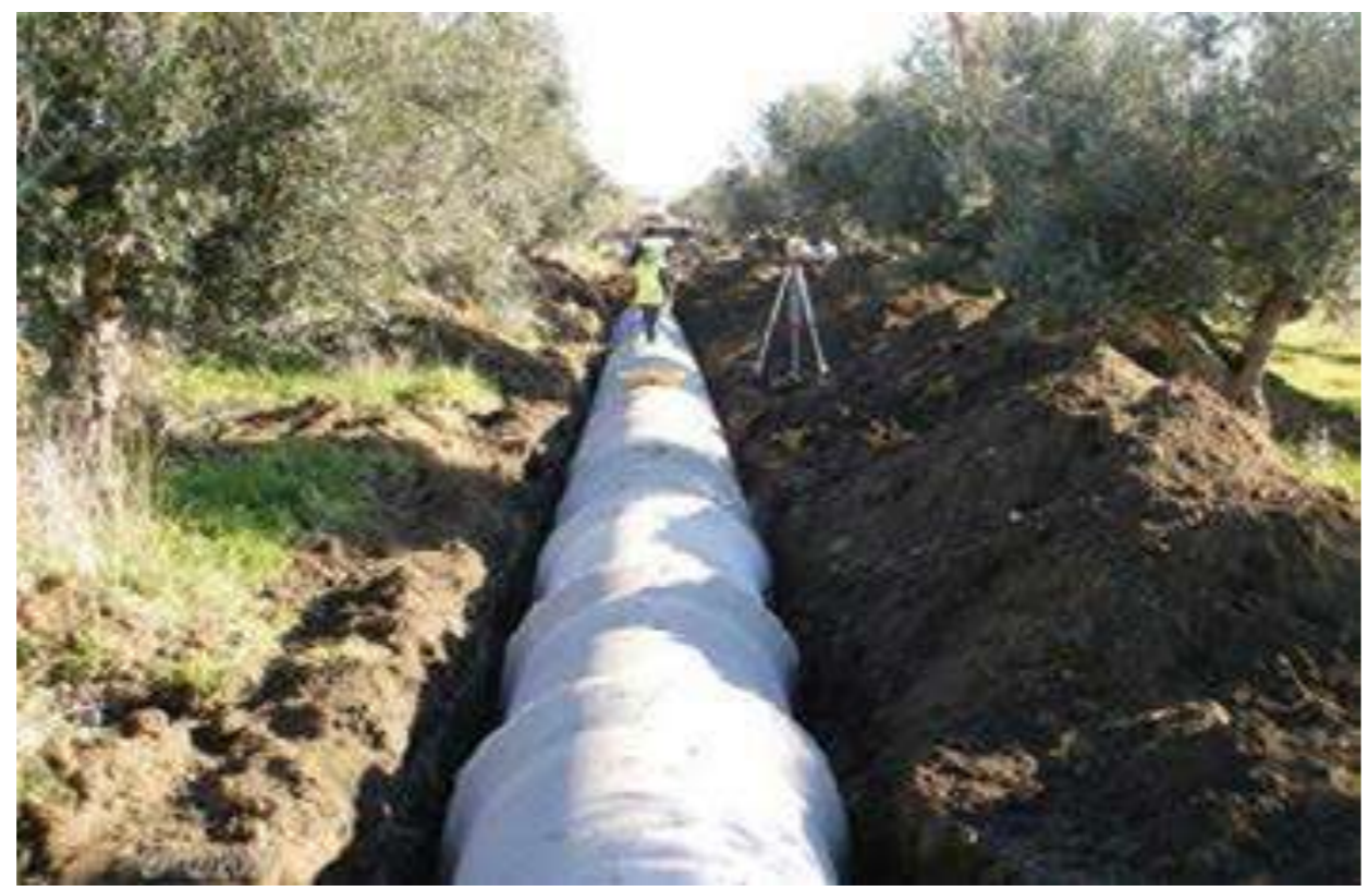
BASIC SANITATION WORKS SOUSEL, PORTUGAL
